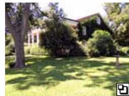
Ivy Covered East Facade
