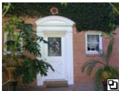
East Arched Entry w/ Gas Light
